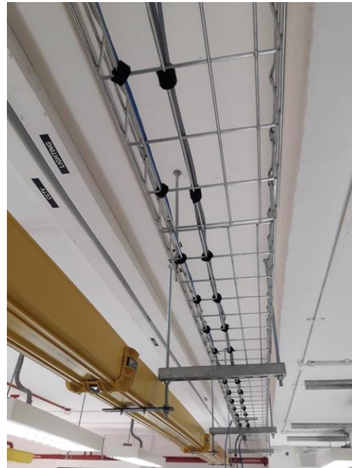
Figure 1.1: Cable grouping based on cable type Figure 1.1: Cables with Velcro at cable basket
