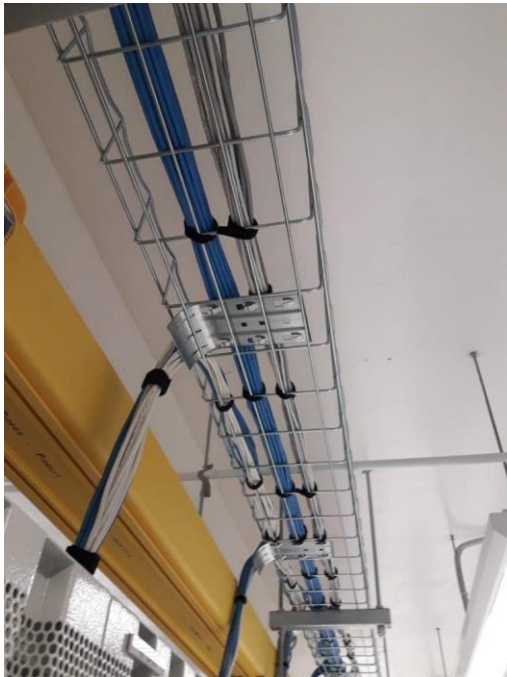
Figure 1.1: Cable grouping based on cable type Figure 1.1: Cables with Velcro at cable basket
