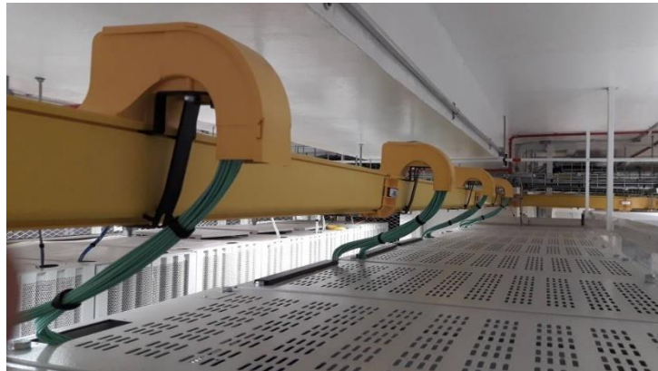
Figure 1.6: Fiber cables organized using Velcro
